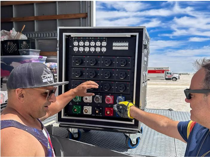
Each of the 50 amp outputs from the distribution box can be fed, via a single 50-amp cable, into a **Spider Box**. A spider box takes the 50 amp cable as input, and contains a whole bunch of household-style electrical outlets that can be plugged into.
